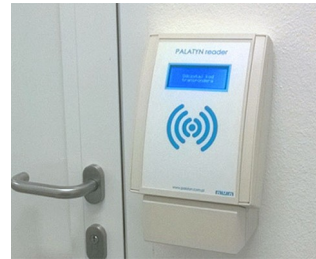
RFID access control readers
