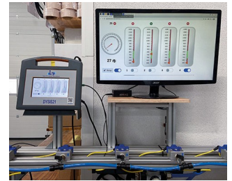
Monitoring system for cleaning nozzles
