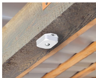
Motion detector with sensor for automatic control
