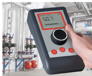
Find compressed air leaks using ultrasound
